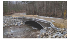
USFS - Sherando Bridge
